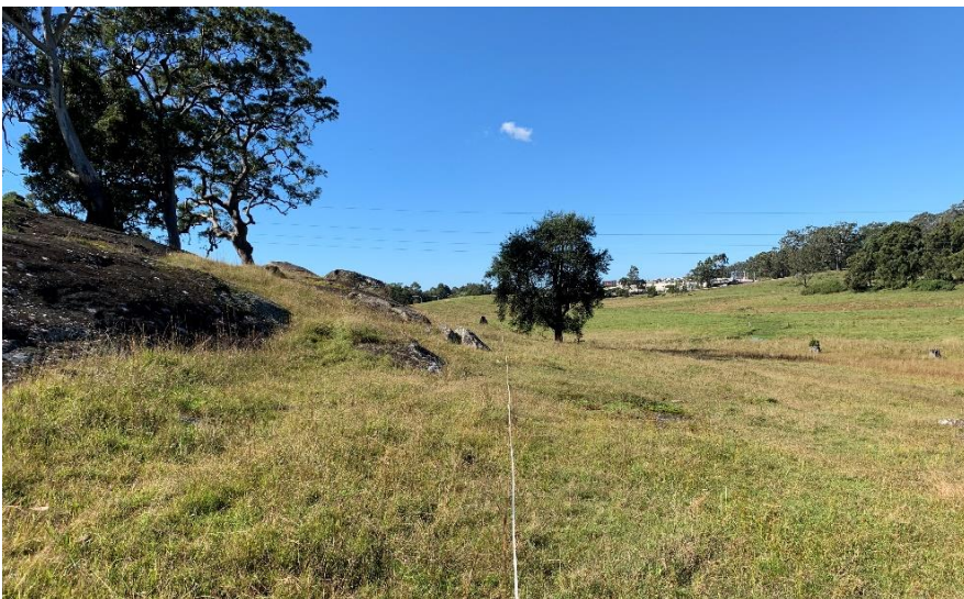
Photograph 3: PCT 684 – low condition
