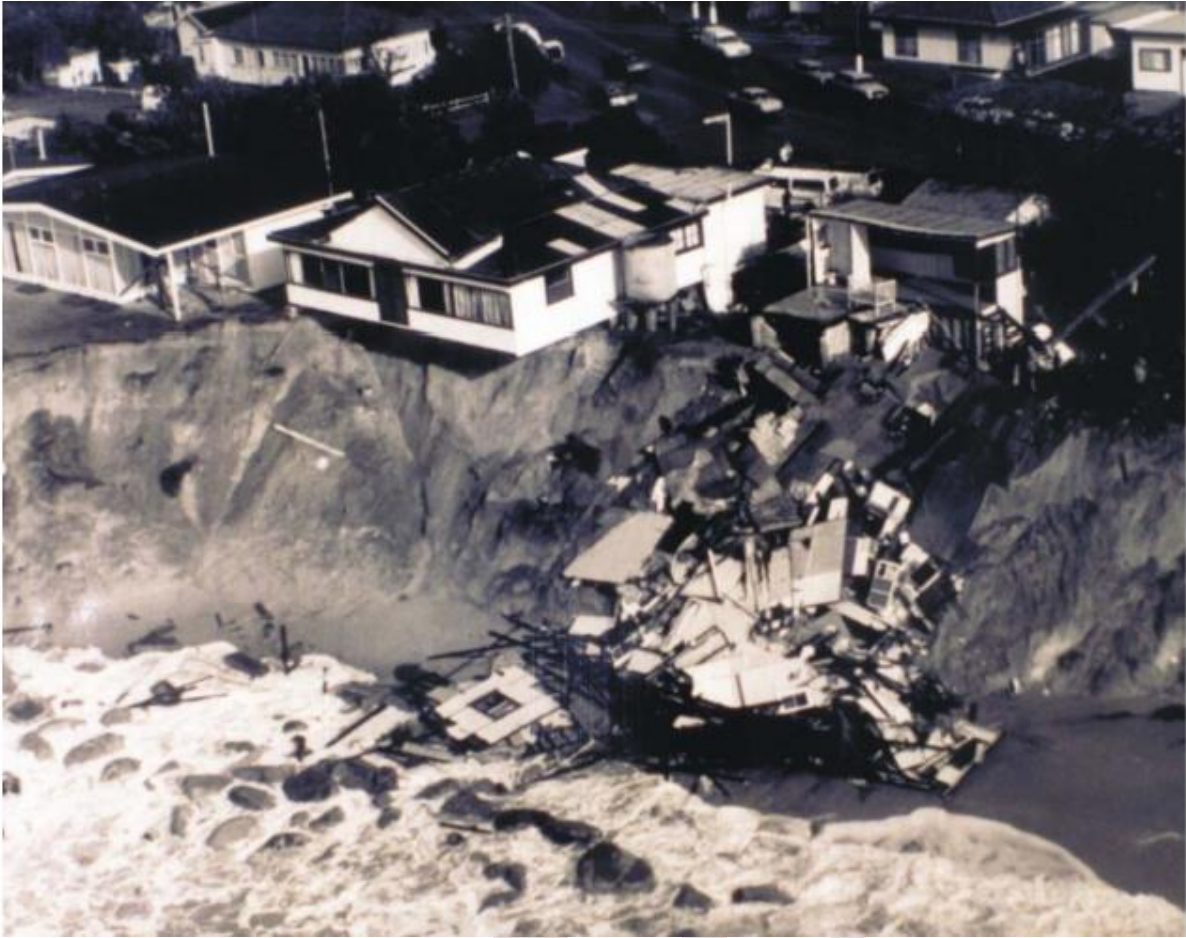
Figure 3.2 Collapse of house at 23b Ocean View Drive Wamberal in June 1978 (News Limited)
